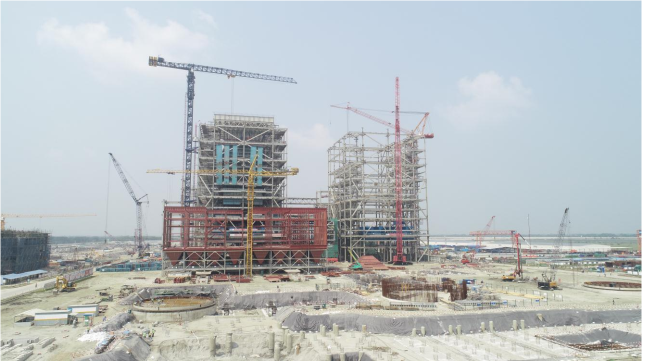
Work Progress of Payra 1320 MW Thermal Power Plant Project (1 st Phase) (Under JVC)
