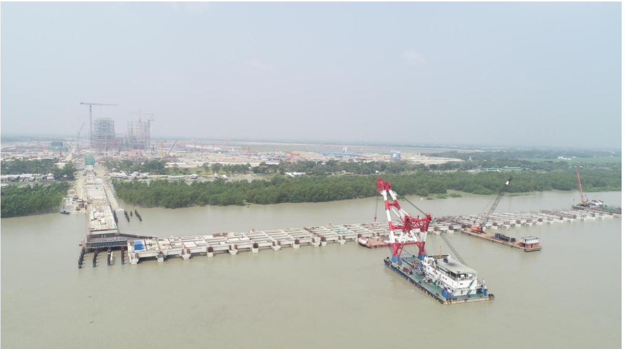
Work Progress of Coal Jetty at Payra 1320 MW Thermal Power Plant Project (Under JVC)
