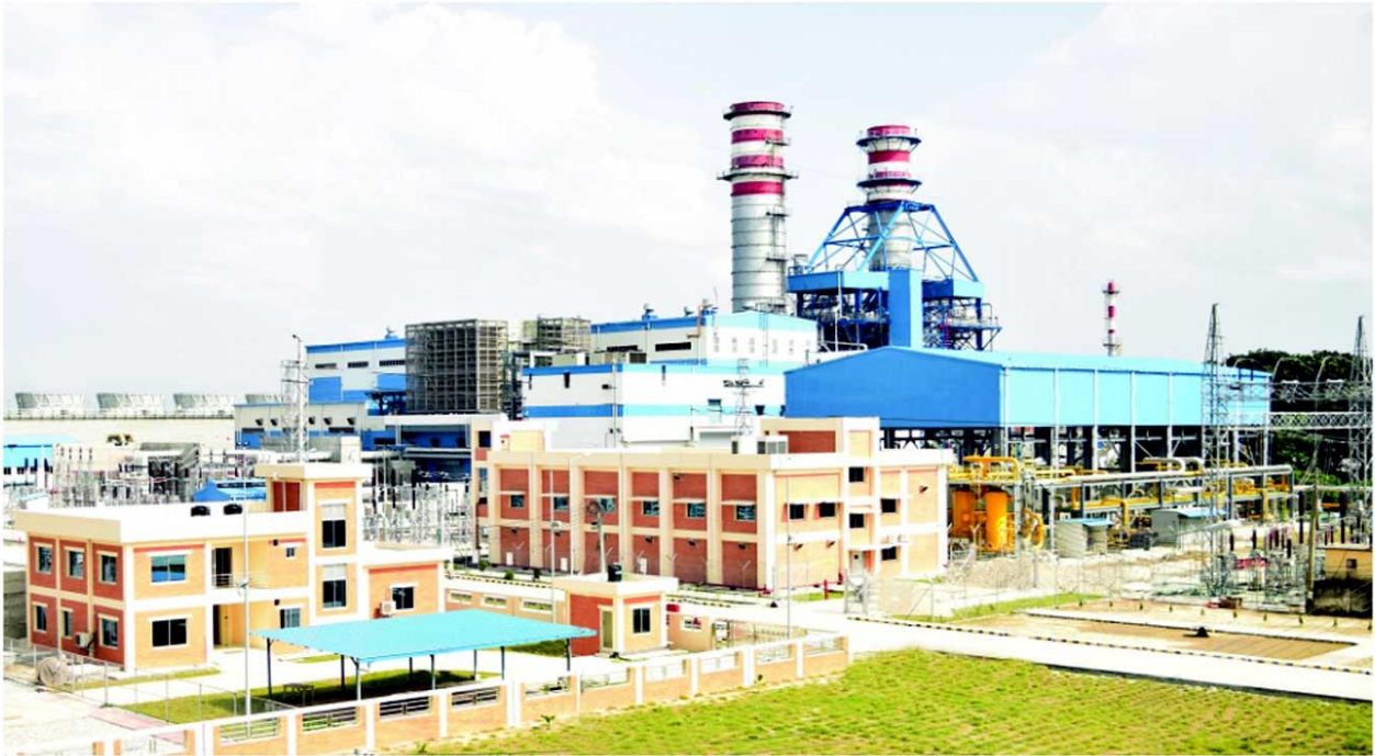
Bheramara 410 MW Combined Cycle Power Plant
