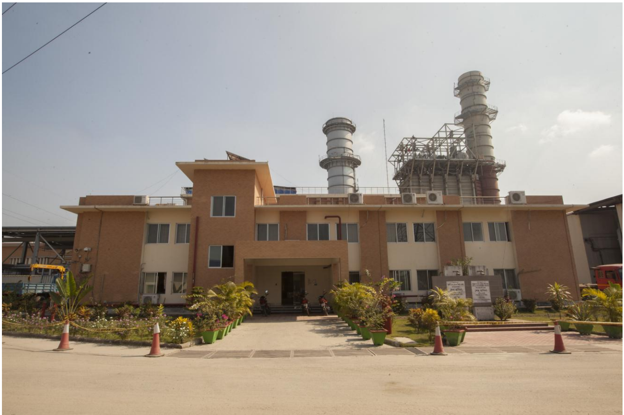
Khulna 225 MW Combined Cycle Power Plant
