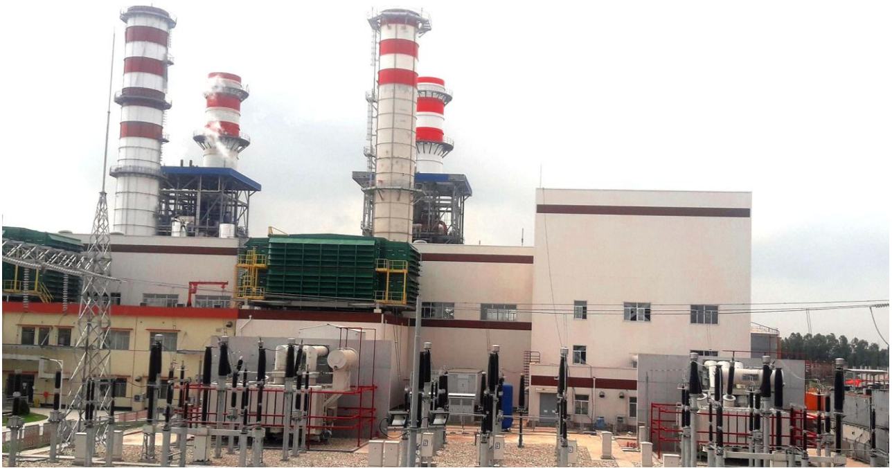
Sirajganj 225 MW Combined Cycle Power Plant (3 rd Unit) (GT)
