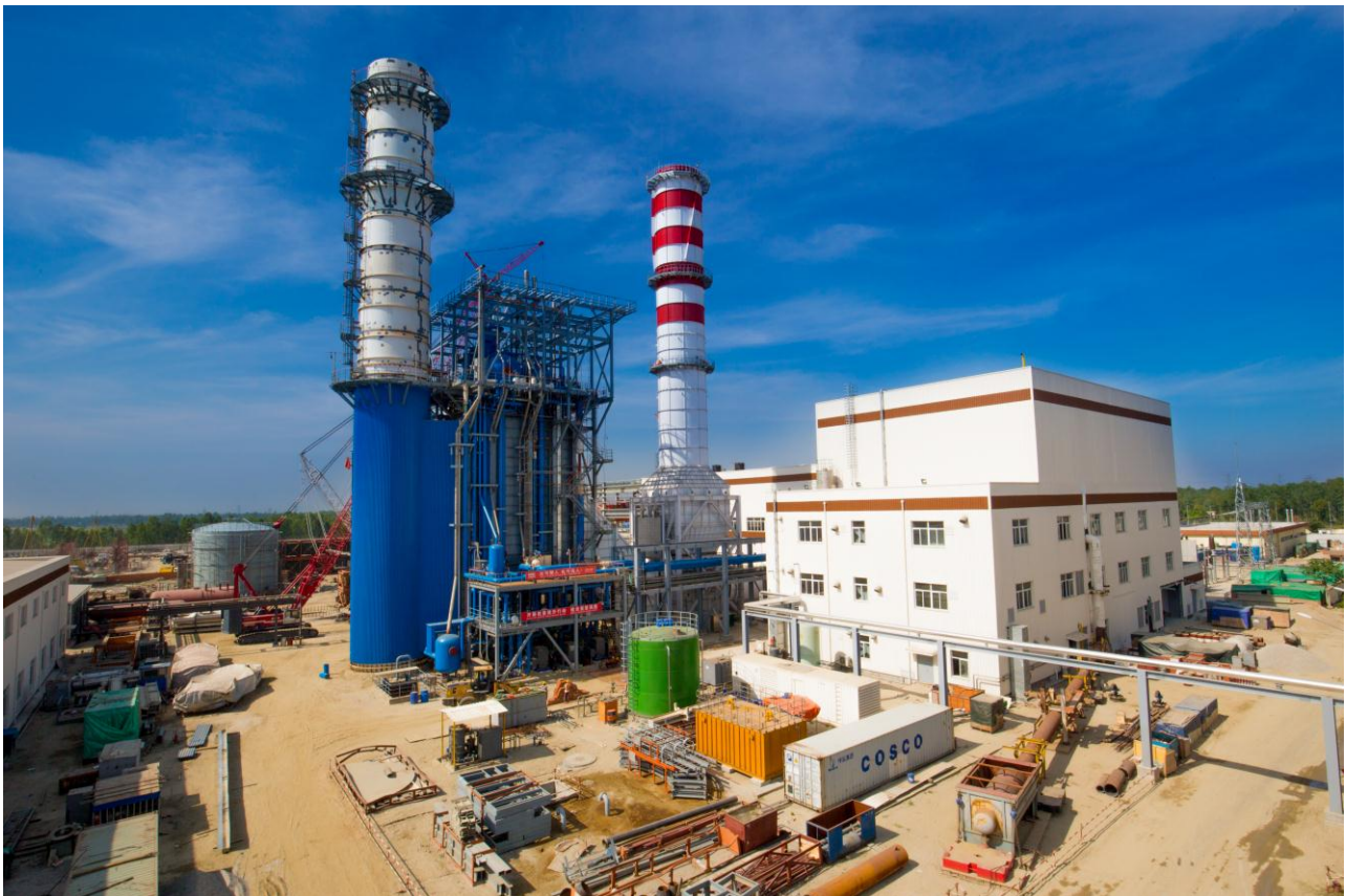
Sirajganj 225 MW Combined Cycle Power Plant (2 nd Unit)
